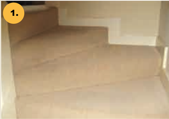
Begin by removing the carpet from your stairs, this will reveal the substructure
