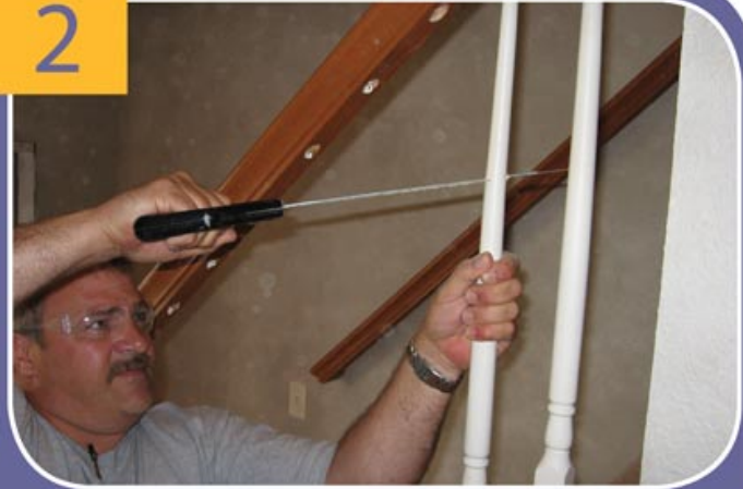
Cut the wood balusters in the middle and discard.
