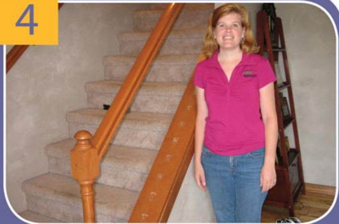
The Staircase with balusters removed.
