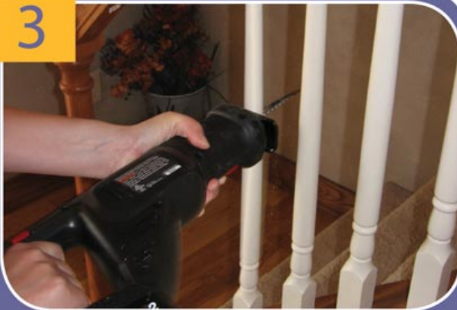
Cutting balusters with a reciprocating saw saves time.
