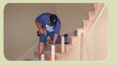
Construction angle brackets from any strong and straight construction material. The angle brackets will have a lot of force against them so take your time and make them very strong. The base that is screwed to the tread should be a minimum 3" wide and 12" long. The vertical should be a minimum of 3" wide and 12" long.
