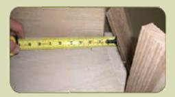
Lay out the location of your handrail and install angle brackets with at least 4 screws into the stair treads. If the handrail is being bent while disposable construction treads are in place, be sure the construction treads are firmly attached. If the angle brackets are attached directly to the final treads, then the holes in the stair treads can be filled and sanded after installation.
