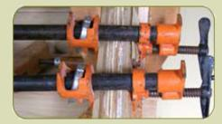
Begin to add clamps working from the center of the bend outward. You may have to loosen some clamps and re-tighten them. Look for consistent and even glue squeeze out along the top of the handrail. Any area that has a crack or uneven glue squeeze-out will need additional clamps. As a general rule, apply a clamp every six inches.
