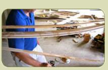
Wet the handrail with water and pre-bend it by placing it against the brackets and clamping it. Wet the bending mold as well so that it will become flexible. If the handrail is being installed around a tight radius then apply several applications of water to make the handrail more pliable. Bend the handrail gently by increasing the clamp pressure over 48 hours.
