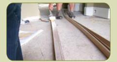
Remove the handrail that has been pre-bent and has a memory of the shape that it will be when installed. Apply glue to the handrail. Place the bending mold on the outside of the handrail. The bending mold will protect the handrail from the clamps and spread the force of the clamps across the handrail.
