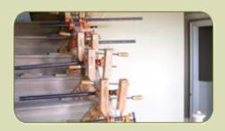
Allow the handrail to sit 24-48 hours before moving the clamps. Plan to spend several hours with a chisel and sandpaper removing glue and shaping the handrail.
